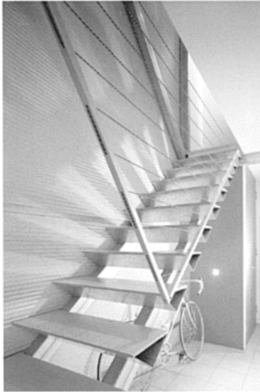
11.6 Clarke McLeod House, Brisbane, 2001: staircase of folded galvanized sheet steel and ply top (stressed skin construction)
