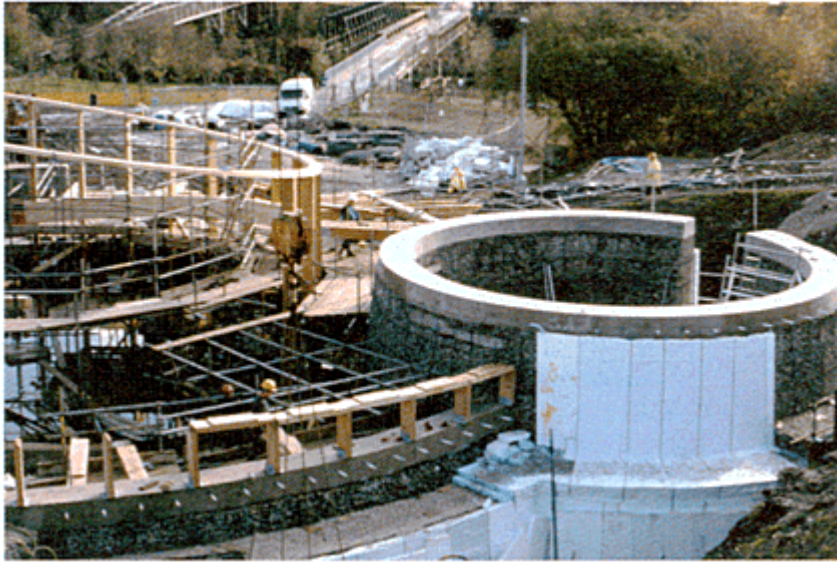
5.15 Trapion walls under construction
