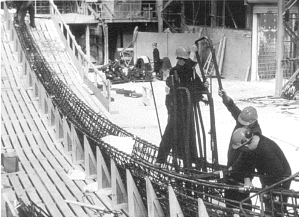
5.10 'Tusk', reinforced-concrete cage fabrication
