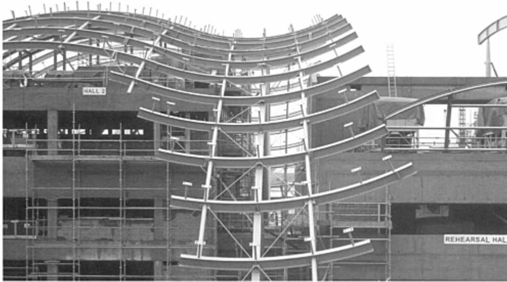
7.13 Detail of the complex roof structure comprising interlocking toroid forms
