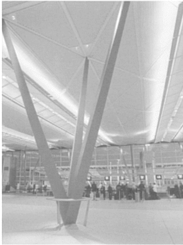
11.12 Tripod columns and shell-truss roof
