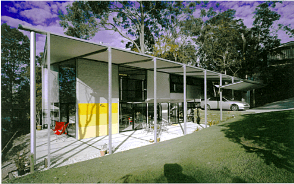
11.4 Clarke McLeod House, Brisbane, 2001: view of exposed structural frame and ‘colonnade’ to north elevation External wall structure
