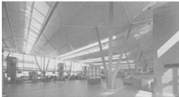
11.13 Walk-through check-in counters with tripod columns
