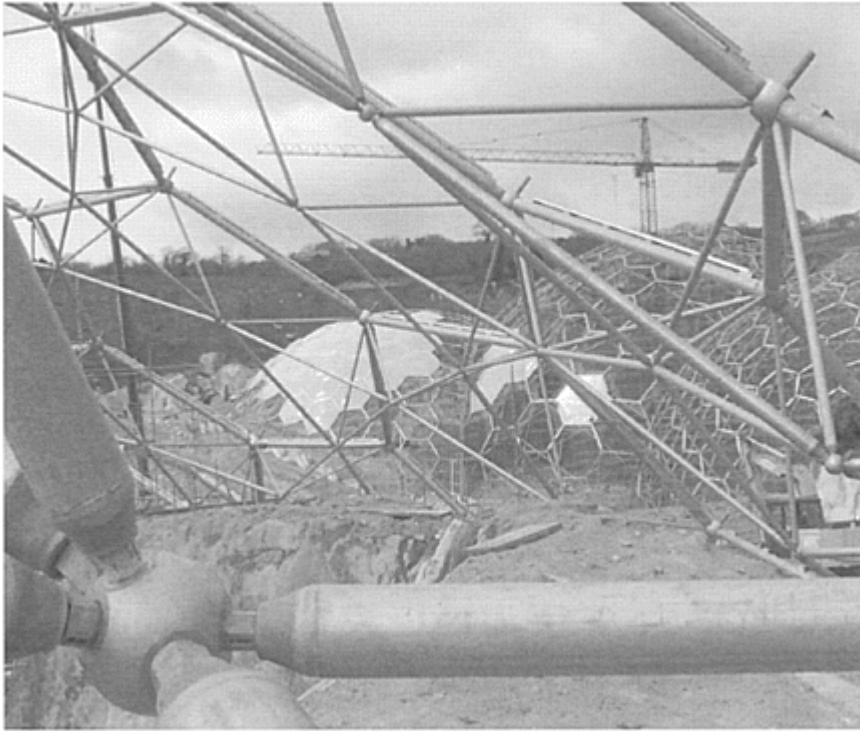
3.20 Eden Project, Cornwall, with Nicholas Grimshaw & Partners, dome structure detail, 2001
