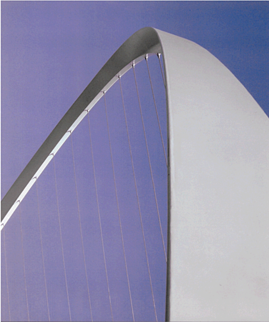
13.12 Gateshead Millennium Bridge, 2001: the constantly changing section of the arch has been designed to catch the light and reduce the structure's visual bulk
