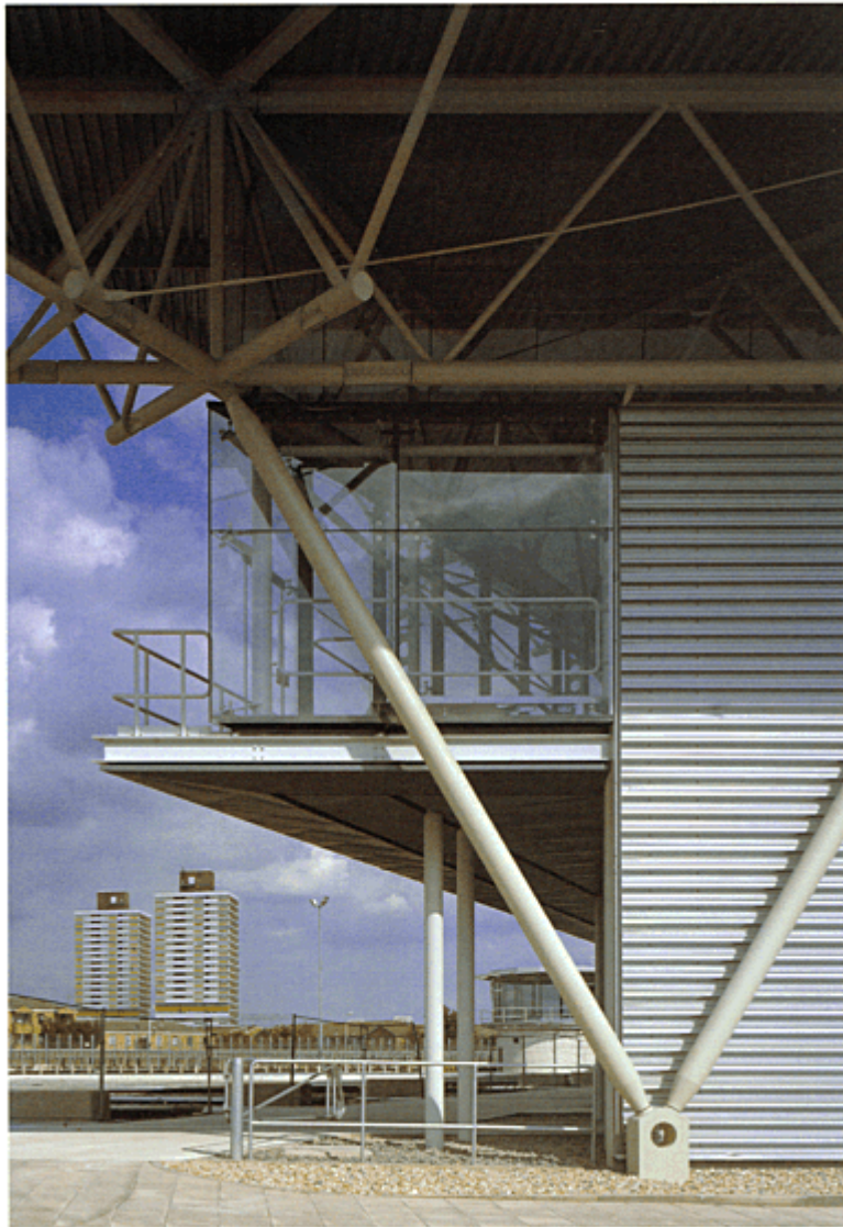
13.13 Stratford Market Depot, London, 1999: the articulation of the structure and materials combined with its acute angle creates lightness
