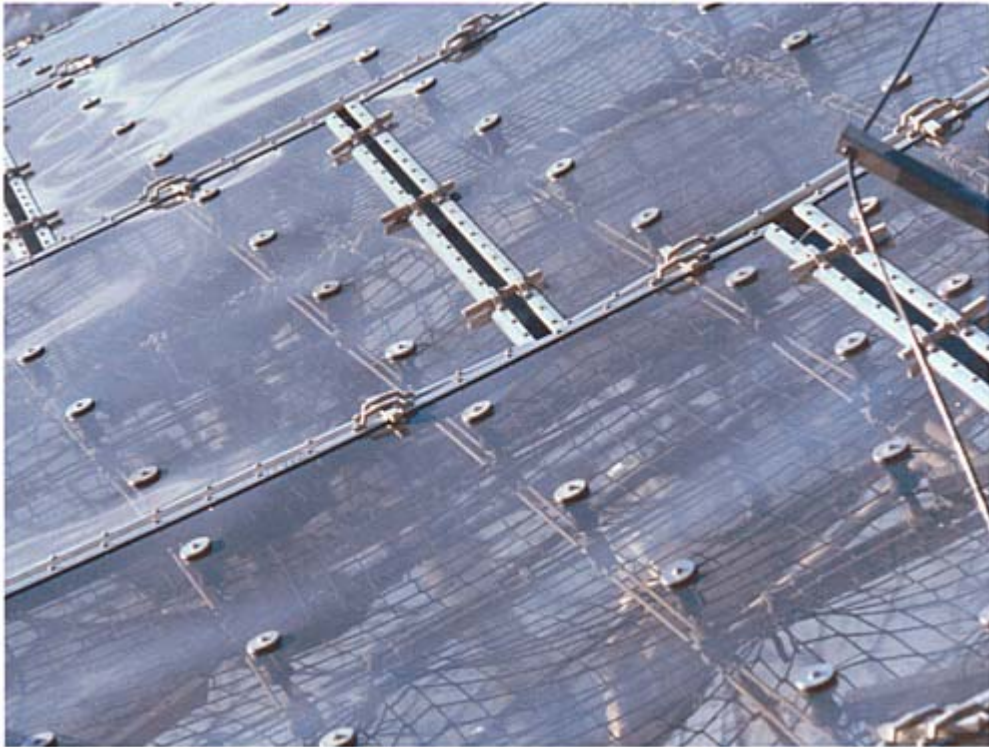
7.2 Munich Olympic Stadium: detail
