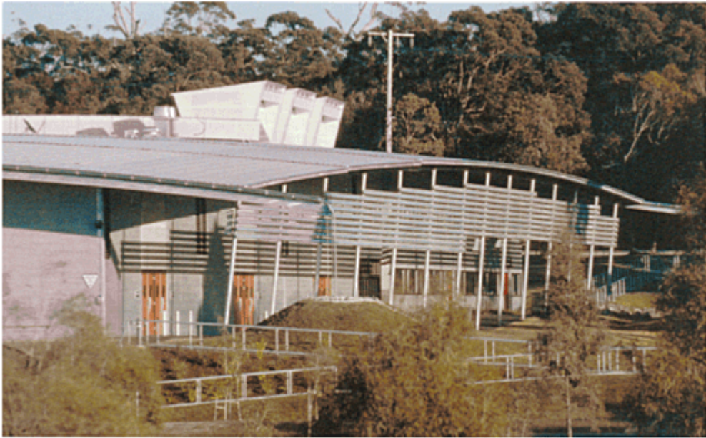
11.14 Sunshine Coast University Innovation Centre, Queensland Australia, 2001: view along the colonnade with thermal chimneys (architect: Bligh Voller Nield)
