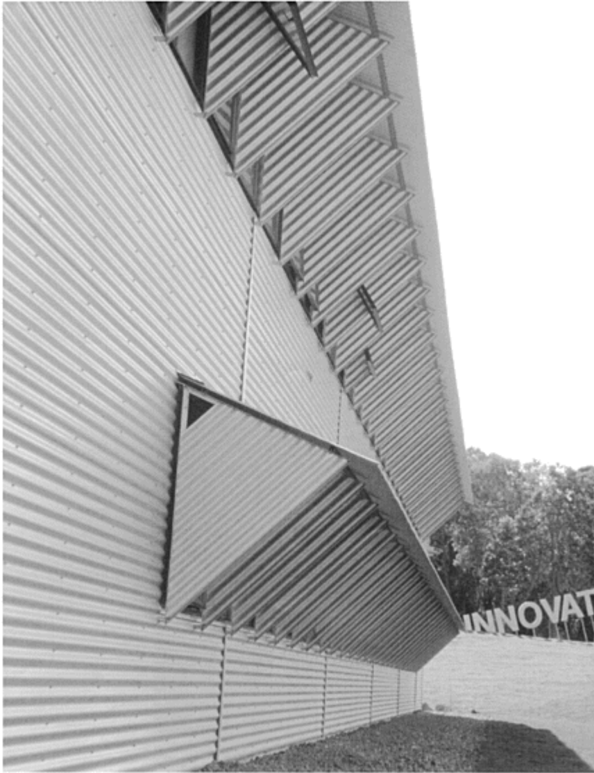
11.16 Sunshine Coast University Innovation Center: cladding and sunshading
