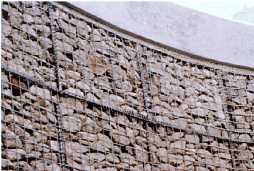
5.16 Completed trapion wall
