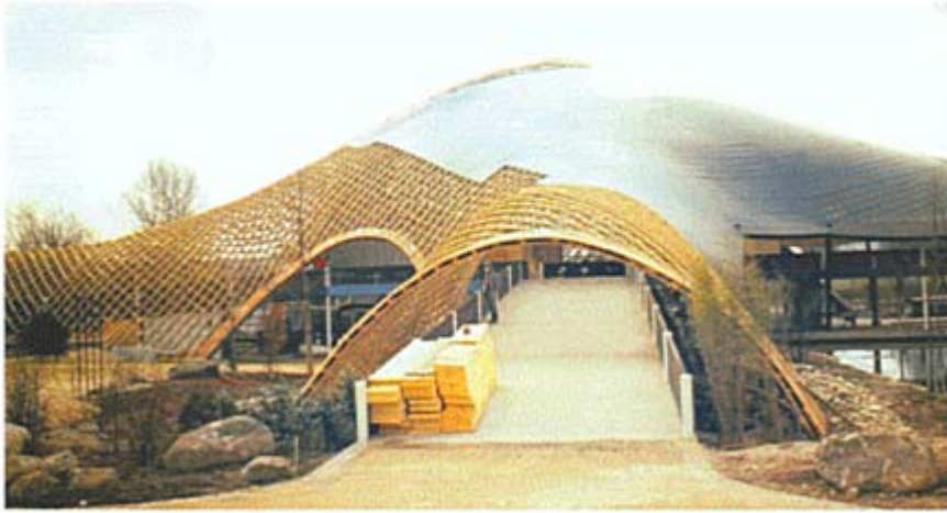
7.6 Mannheim Bundestgartenshau, Germany, 1975; a translucent shell created by a timber lattices framework and clad in PVC coated polyester
