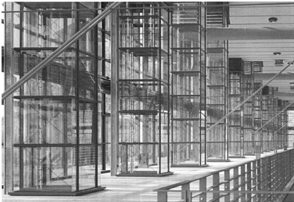
12.3 Hanover Trade Fair Hall, 2000: glass ducts for air circulation
