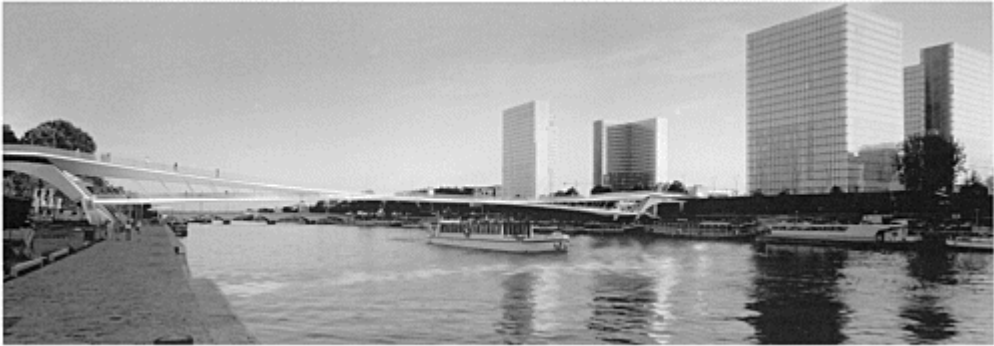
13.10 Bercy Bridge, Paris, 1999: competition entry for a 200-metre-span footbridge over the Seine with 180-millimetre cables
