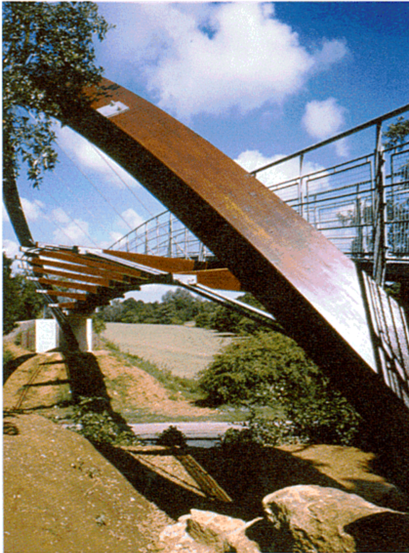
5.8 A4 Millennium Bridge, UK, 2000
